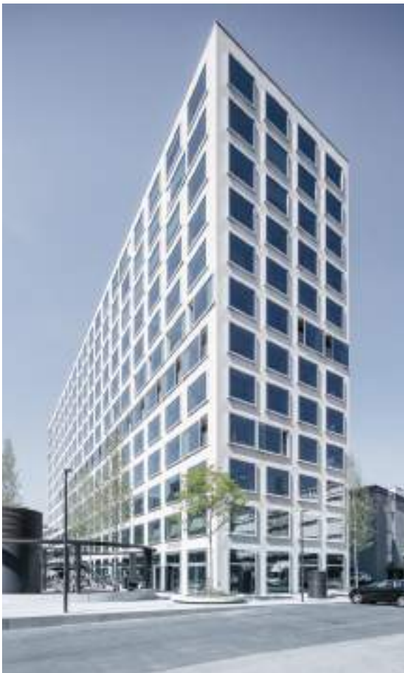
Diakonie Bethanien, Zurich Height: 40 m Sliding units: 500 Project: complete façade cladding
