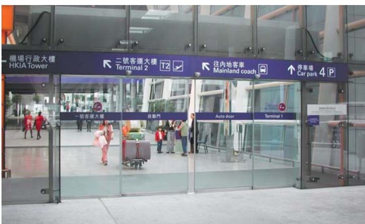
▲ Hong Kong International Airport Sliding door SLM - 1 -Booster (Customized Solution)
