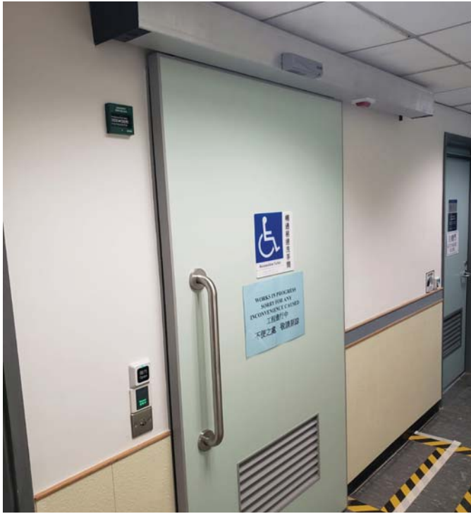
▲ Hong Kong Baptist University Barrier Free Access Solution with Sliding door Operator
