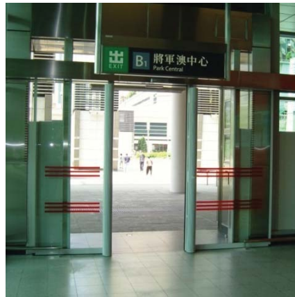
◀ MTR Tseung Kwan O Station SLM-Dual with PS90 Profile System
