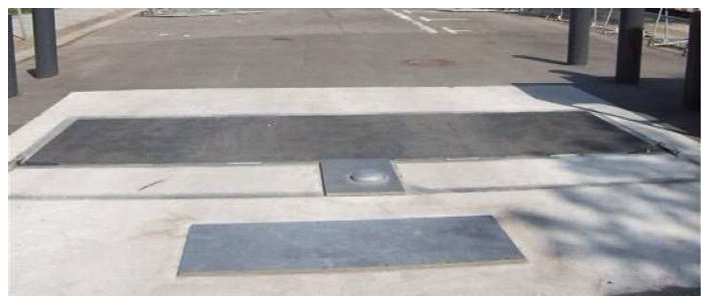
Barrier: barrier is flush to the surface of the roadway in closed position. In opening position: standard height 35 inches (900 mm).
