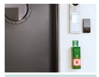
**Escape door terminal:** Safely locked in everyday use while allowing quick and easy opening in the case of an emergency. These are the most important requirements for doors in escape and emergency routes. Electronic escape route securing systems assist in fulfilling these apparently contradictory requirements.
