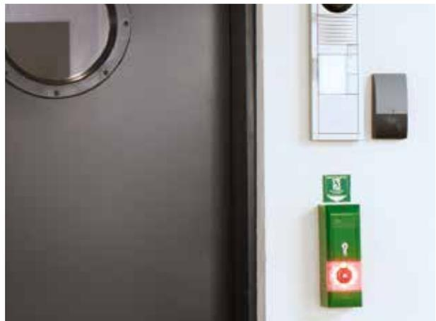
**Escape door terminal:** Safely locked in everyday use while allowing quick and easy opening in the case of an emergency. These are the most important requirements for doors in escape and emergency routes. Electronic escape route securing systems assist in fulfilling these apparently contradictory requirements.
