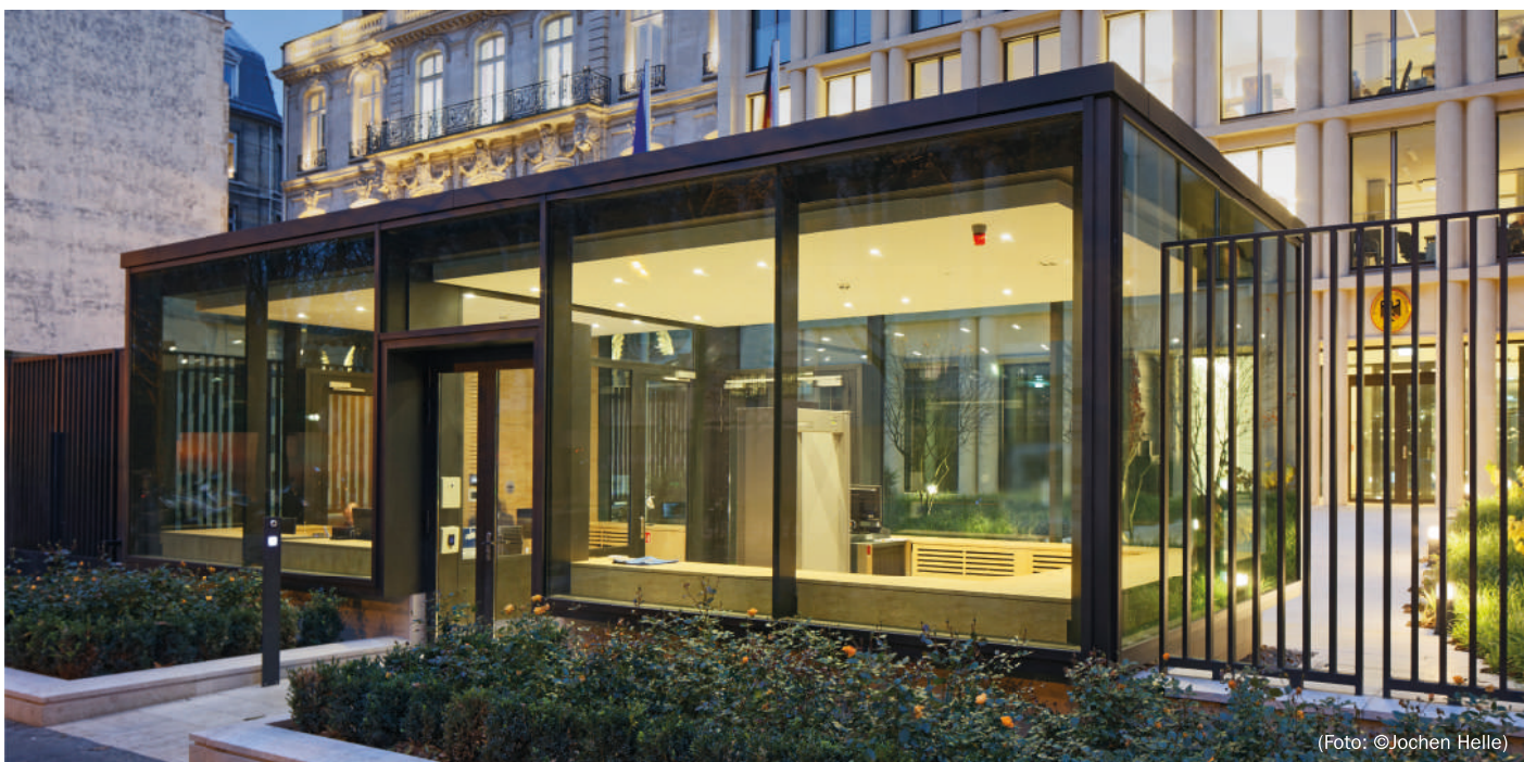
A fully-glazed, cube-shaped guardhouse for a German Embassy abroad with a security facade made from box profiles and an aluminium add-on construction, which is able to bear the 2+ tonne weight of the 4.6 x 3.2 m individual security glazing with ease.
