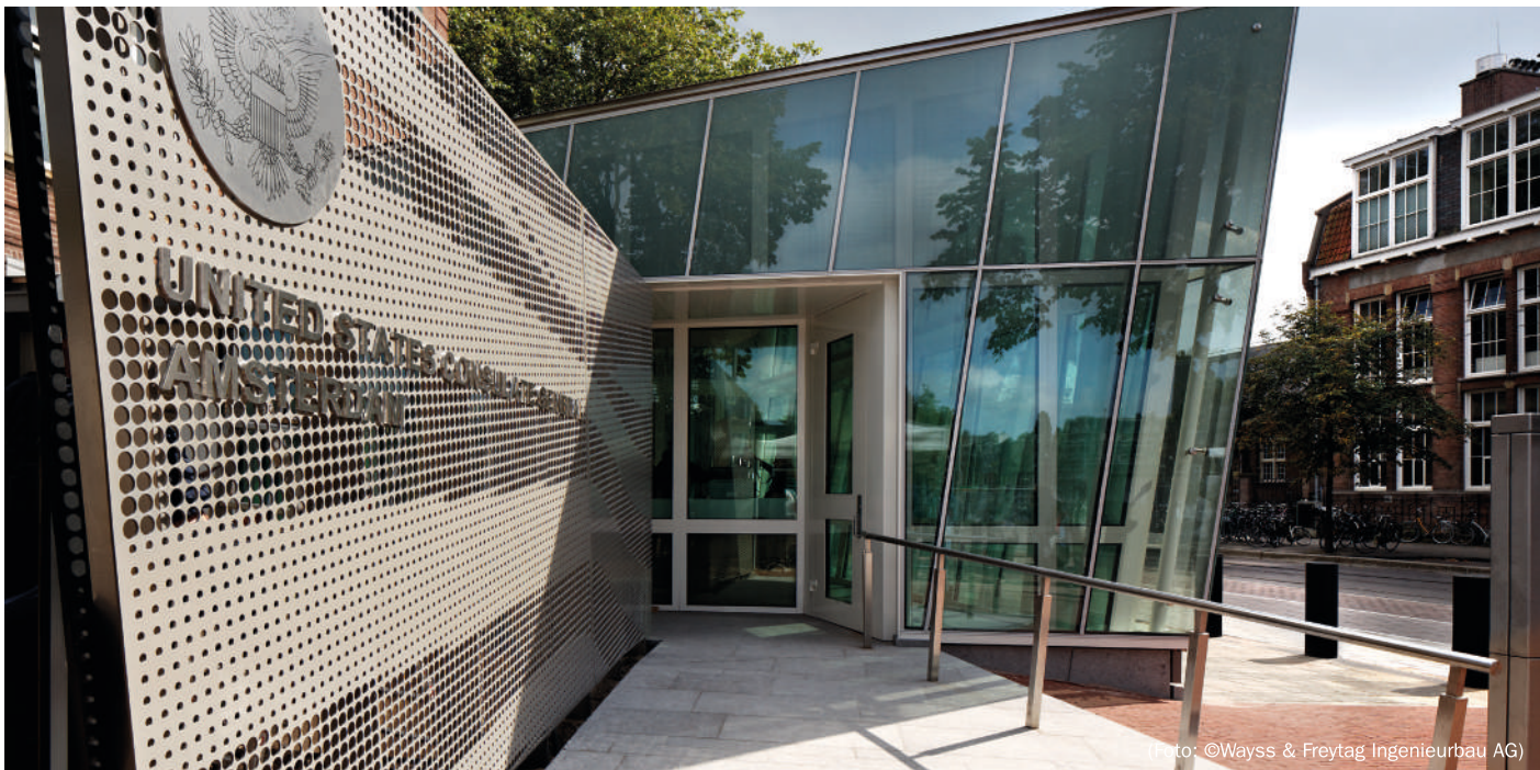
Generous glazing of the guardhouse for an American property with a sloping double facade and roof construction. All of the components were security-tested in advance in accordance with specifications of the US Department of State.
